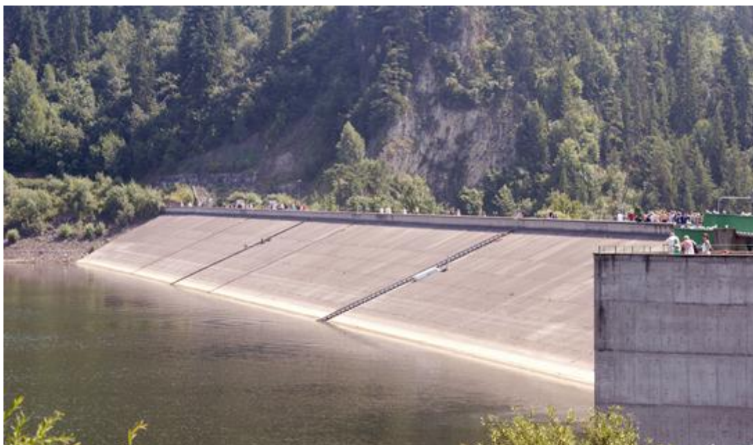
Fig. 2. View on the riverside embankment from the side of Lake Czorsztyńskie, with a visible walkway
