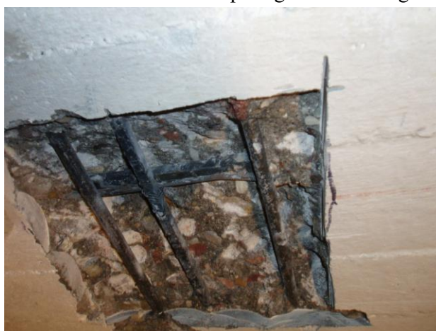
Fig. 4. Inspection hole of the cold storage building's ceiling in Wloclawek.
