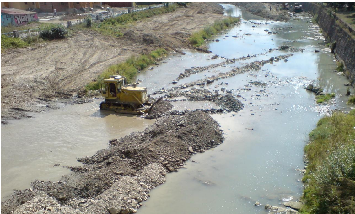
Fig. 2. Initial works in the Kamienica riverbed in Nowy Sącz in 2009.
