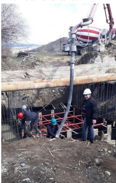
Irrigation System Rehabilitation Process, Skhvilisi
