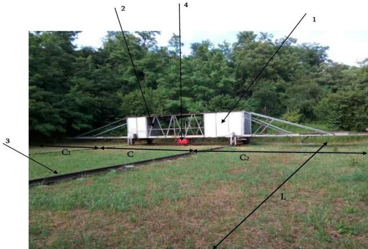
Photo -1 Bridge assembly
