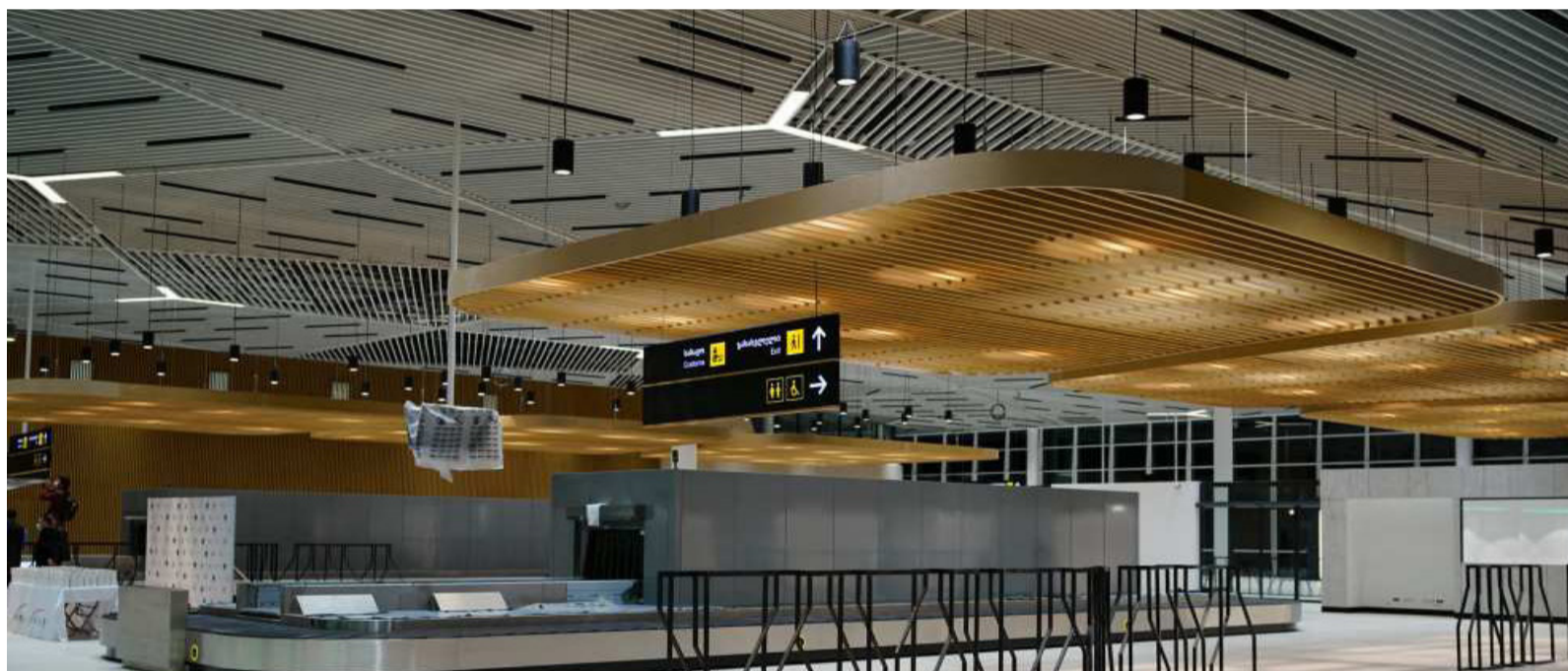
► The expansion project of the airport started in November 2017 with an investment of €10 million.
