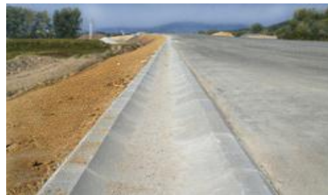
Figure 5. Construction of near-edge water removal chute used in Poland [4, 5]
