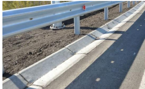
Figure 4. Construction of near-edge water road removal chute used in Russia [2, 3]
