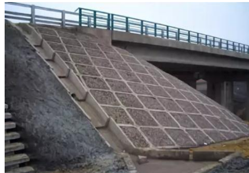
Figure 8. Roadway telescopic chute B -7 used in Russia [8, 9]
