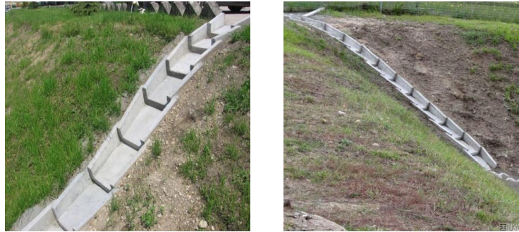
Figure 11. The view of telescopic slope water diversion chutes used in Poland and Germany [14, 15]
