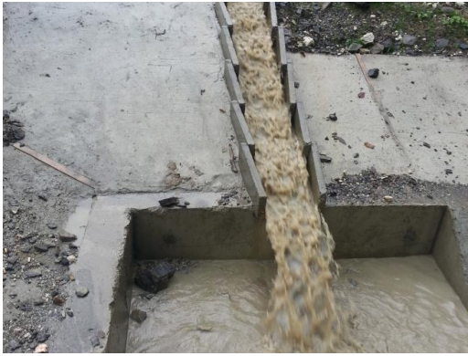
Figure 12. Photograph illustrating the nature of the water flow in telescopic chute [21]
