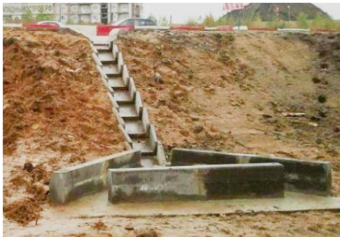
Figure 8. Roadway telescopic chute B -7 used in Russia [8, 9]
