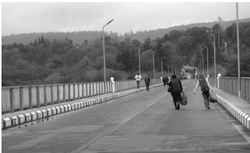
Picture N1 The Ruckhi (Otsartse) Bridge
