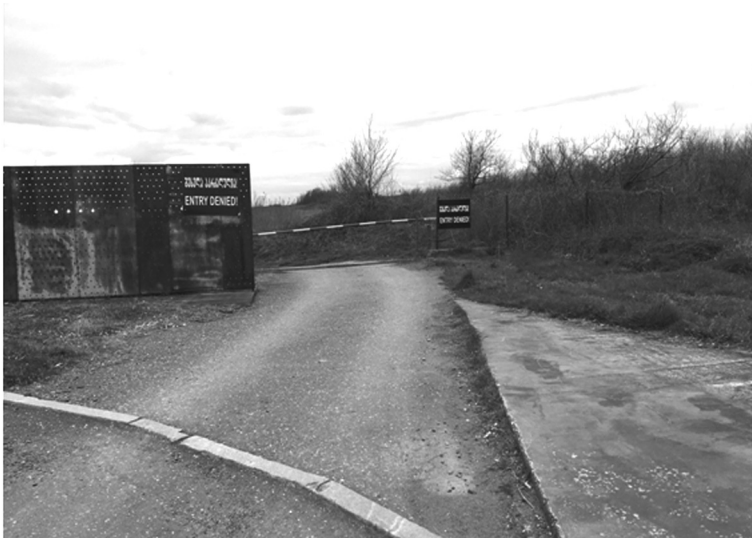
Picture N3 Ganmukhuri-Pichori closed Crossing
