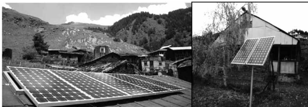
Figure 14. Examples of solar energy use in Georgia
