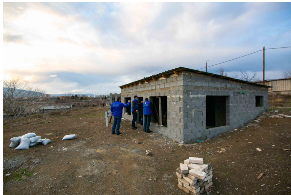
According to PHR, the family was given until December 20 to leave the house
