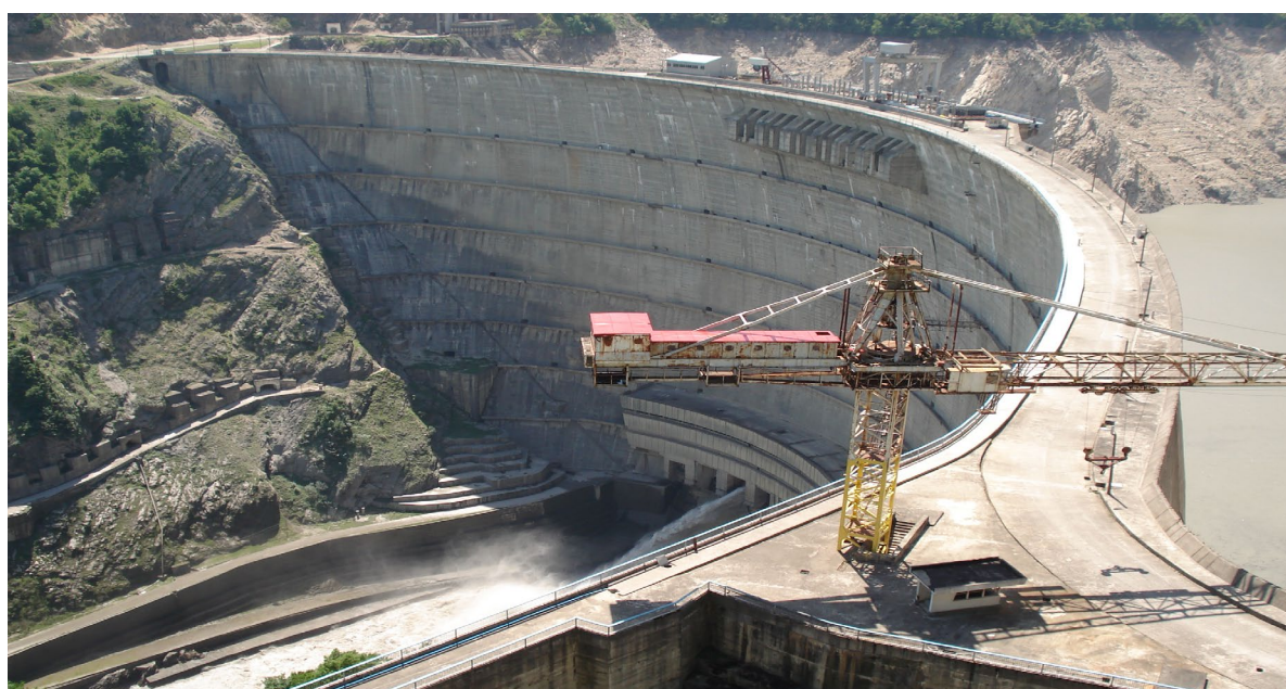
► As a result of renovation works, the volume of water leaked from the tunnel has been significantly reduced.
