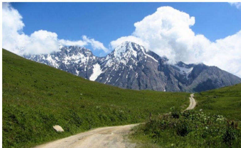
► Reconstruction of Lentekhi-Mestia road will reduce travel time and provide safe and comfortable movement for the local population as well as tourists.
