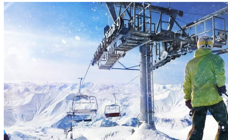
► Rehabilitation of Tetnuldi ski resort will start this year and will cost €5 million in total.
