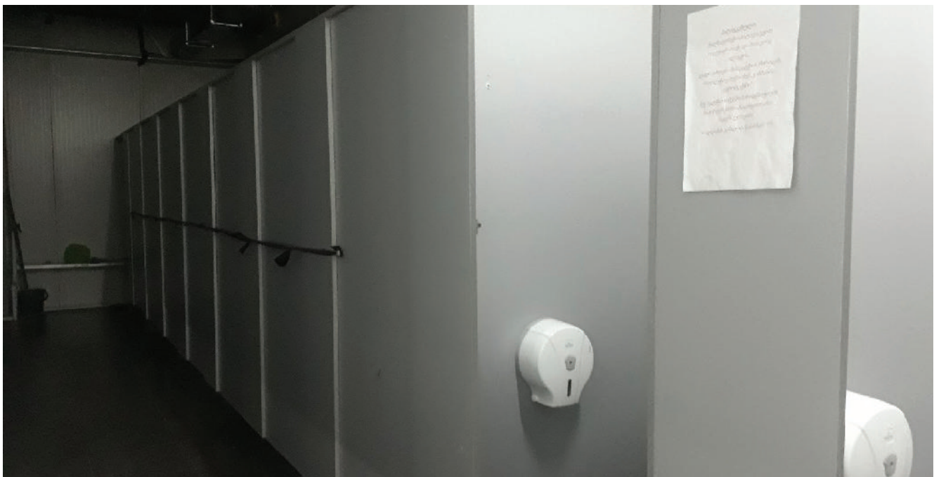
Most of the toilets are locked and none of them have toilet paper. Photo: Tamuna Chkareuli.
