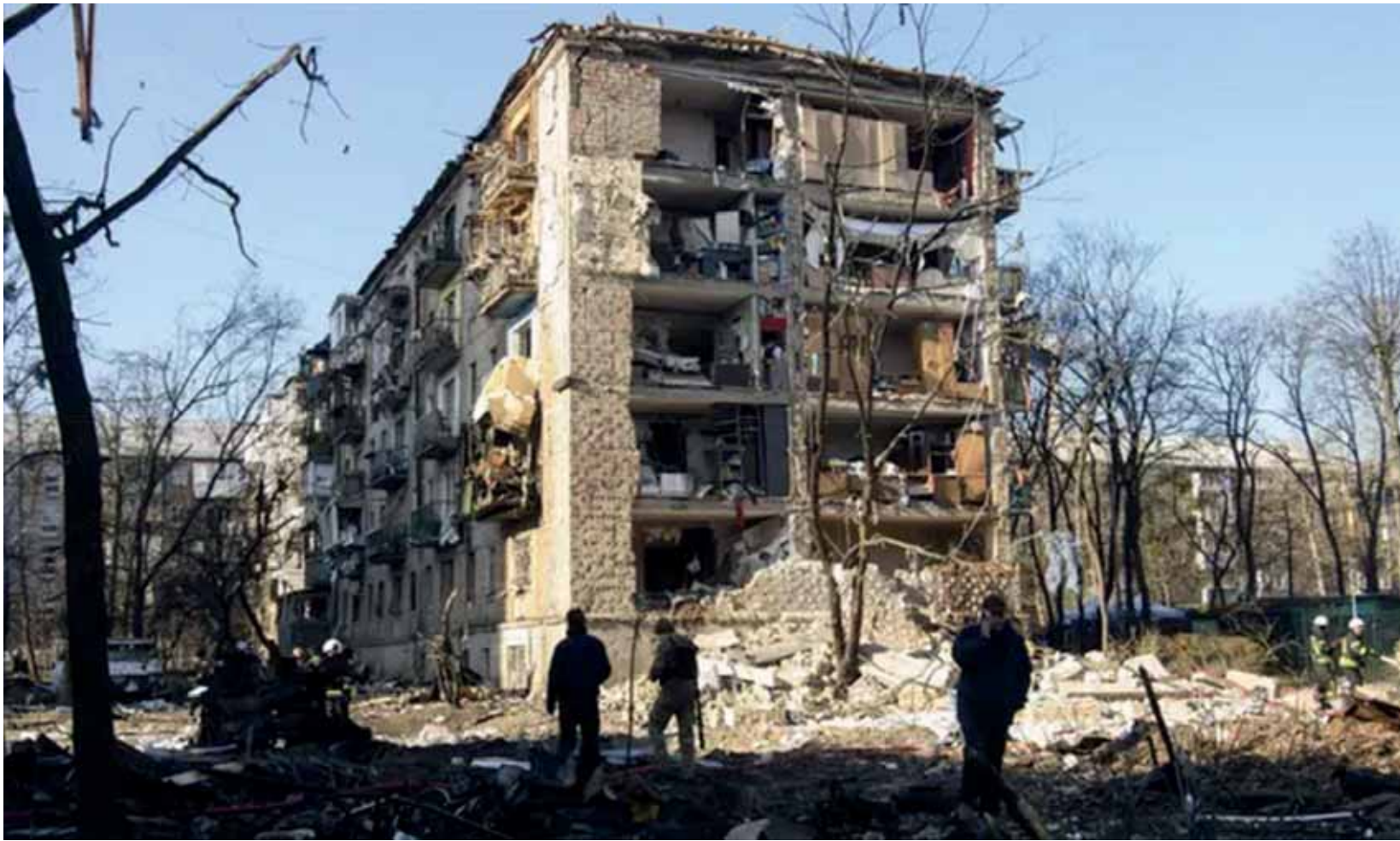
Ukrainians beside a building hit by Russian shelling in a residential area of Kyiv. By Vladyslav Musiienko/UPI/REX/Shutterstock
