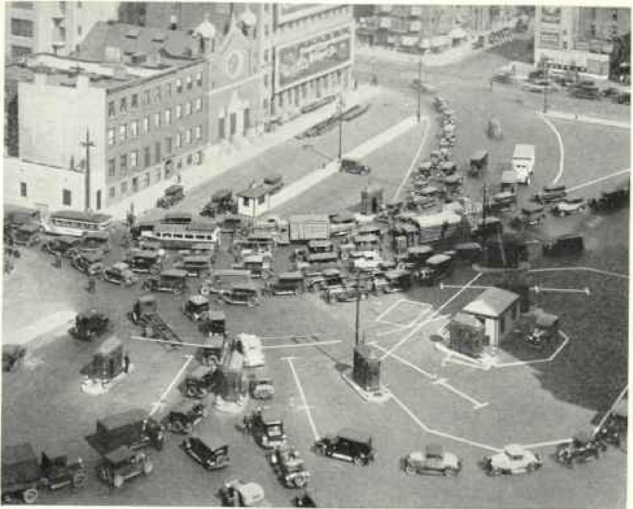
Photograph from Port of New York Authority
