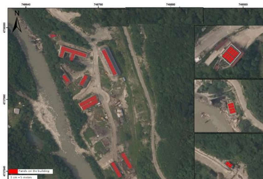
Fig. 5. Solar panels on buildings
