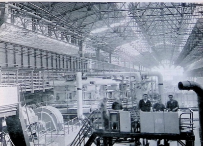
32 The tube-works at the Transcaucasian Metallurgical Works, Rustavi
