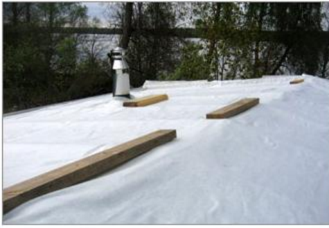
Photo 8. Root protective layer
