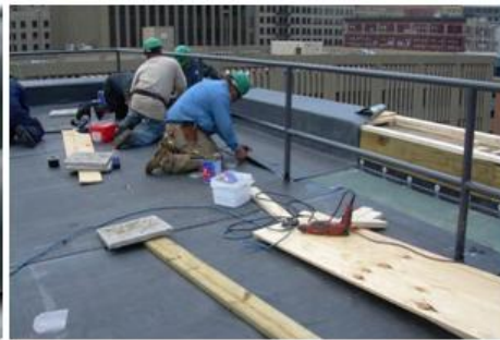
Photo 10. Polymer waterproofing membranes on bitumen base
