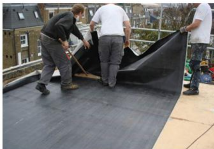
Photo11. Polymer waterproof membrane arrangement on the synthetic base
